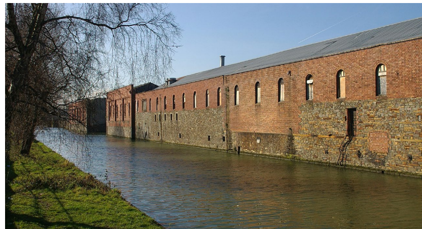
Figure 31 River Avon (above), Feeder Canal (below)
