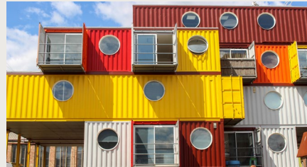
Shipping container offices
